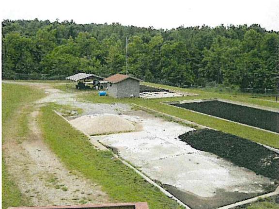
Bed No. 2 remains as originally constructed. Bed No. 3 was improved in 2003 with a polymer system and tractor skids.
