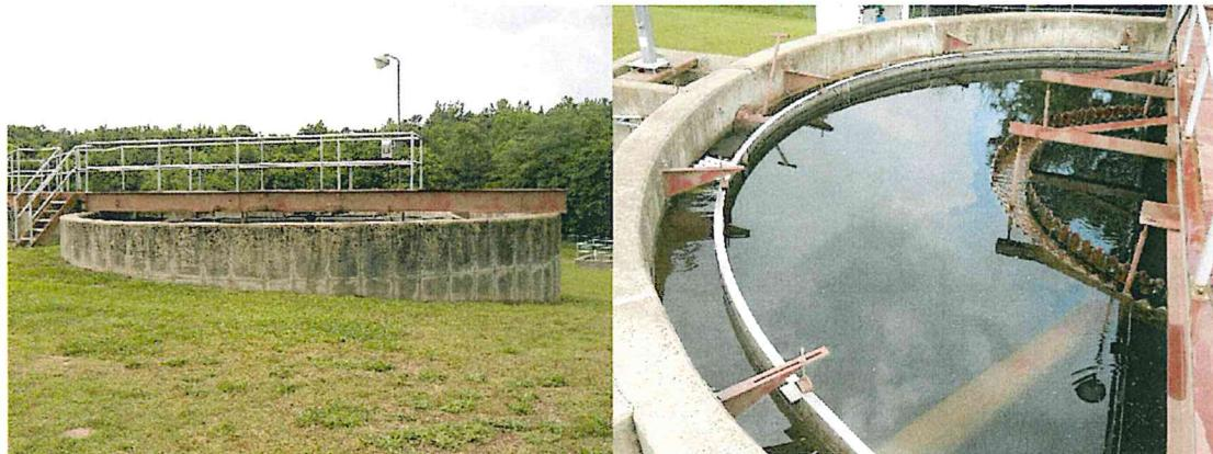
Secondary sludge is decanted from the secondary clarifiers through sludge piping connected to the bottom hoppers. Through a series of valves & yard piping, the operator may select to direct wet sludge to either a tank truck or to one of two drying beds. The preferred disposal method is bay drying; the tank truck is only used when weather conditions prevent drying beds from working effectively.
